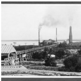
General View of McLachlin Bros. No. 4 Mill
