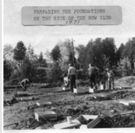
Preparing Club House Foundations
