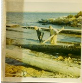
Removing Railway at Bell Park Launching
