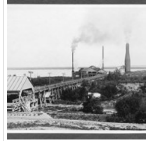
General View of McLachlin Bros. No. 4 Mill
