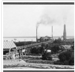
General View of McLachlin Bros. No. 4 Mill
